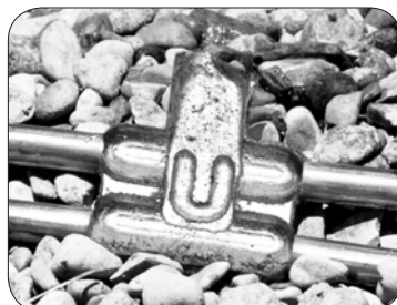
A completed UltraShot connection
