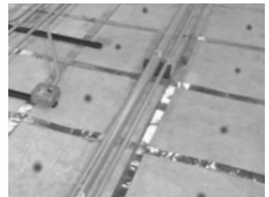
Pedestal locations marked by the dot
