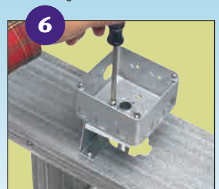
Attach 4x4 metal box to the stand-off bracket with screws (not provided) through pre-drilled holes in bracket.
