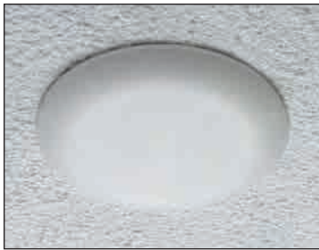
Mounting screws are invisible on the ceiling
