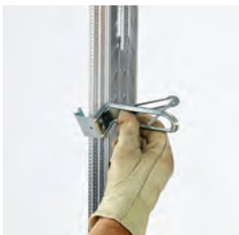
Push support onto stud
