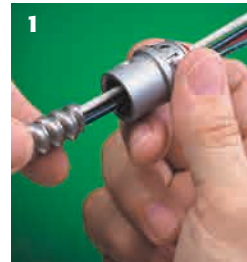
1 Snap fitting onto cable... twist clockwise
